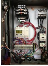
Front opening control panel eliminates the need for 48" side clearance as required by NEC<sup>®</sup> standards.
