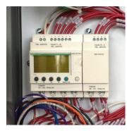
If there is an attempt to override the interlocks; the panel box features a programmable "smart" relay control system that disables the baler. The relay add diagnostic and trouble-shooting capabilities.
