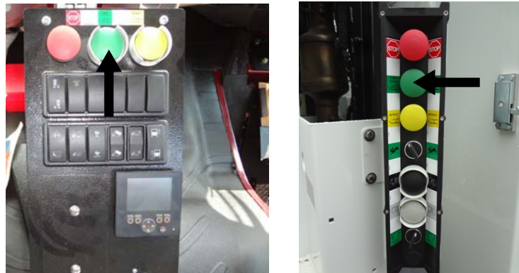
Figure 7-9 Start cycle button: on the control panel (left), on the packer control station (right)
