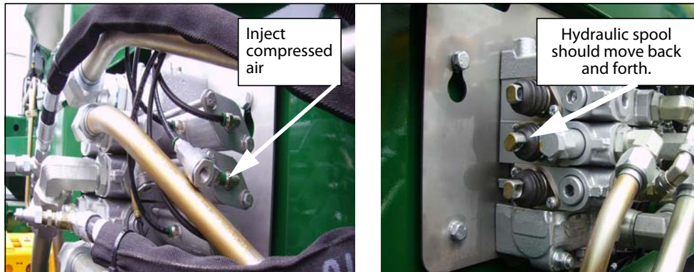
Figure 8-7 Injecting compressed air
