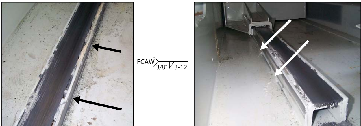
Figure 3-46 Welds on both sides of floor guide
