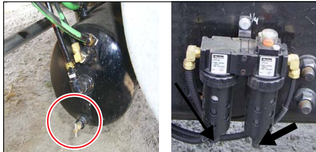
Figure 2-6 Drain valve on air tank (left) and water trap (right)
