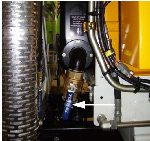
Figure 2-13 Main valve (ball valve) on suction line
