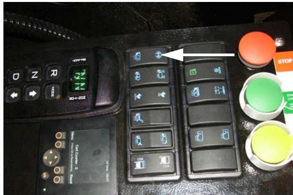
Figure 2-14 Hydraulic pump switch on the multiplexed module
