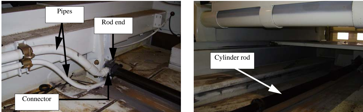
Figure 3-5 Packer hydraulic system
