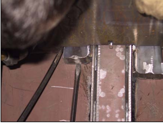
Figure 56. Use pry bars to place the sliding shoe correctly
