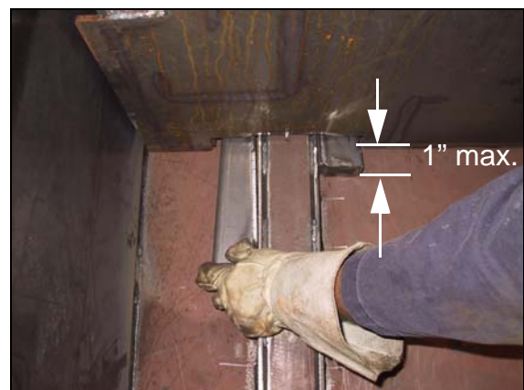
Figure 55. Insert sliding shoes on each side of both rails
