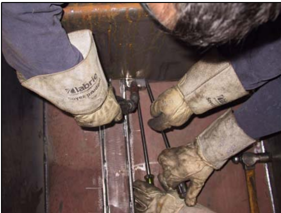
Figure 57. Tack weld the sliding shoe
