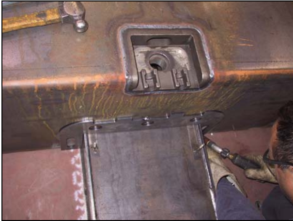
Figure 66. Tack weld the scraper in place
