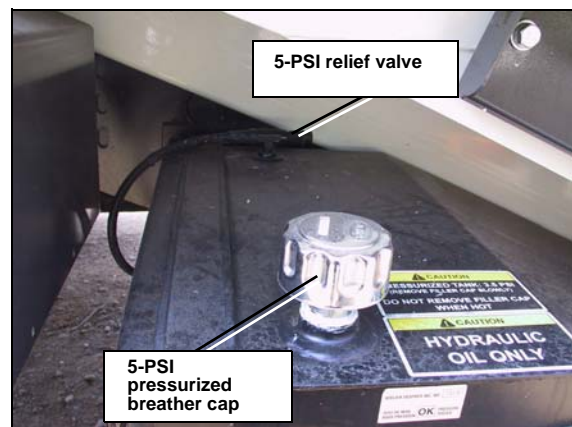
Figure 115. Tank relief valve and pressurized cap
