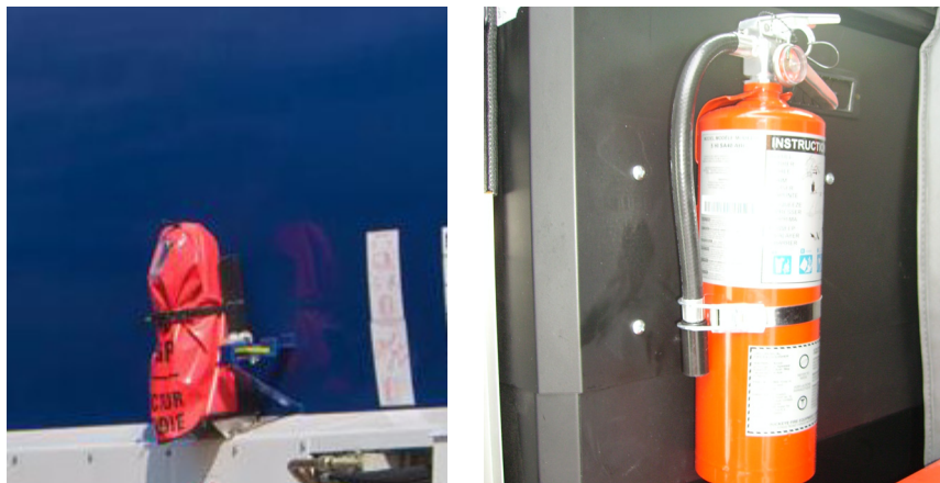
Figure 2-1 20-lb fire extinguisher (left); 5-lb fire extinguisher (right)
